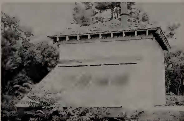
Solar composting toilet on Gallops Island, destroyed by fire in 1982
